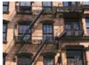
fire escape požarne stepenice
